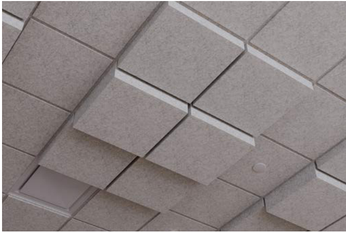
Vista, Box Ceiling Frames in Milkyway
