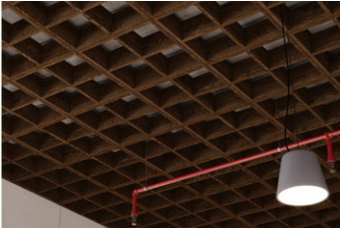
Woven, Windowpane Ceiling Frames in Scorched Timber
